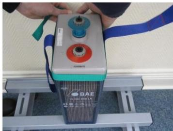
Remove the strap after moving and final stabilized cell position.
