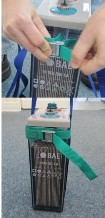
Lead the green strap through the buckle and fasten it tight. Ensure the right direction of the protective strap between cell and buckle.
